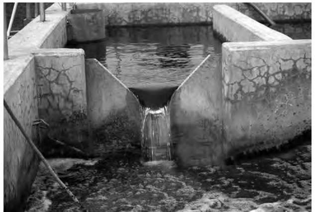
V-Notch installed in the tank's channel to measure the discharge rate
